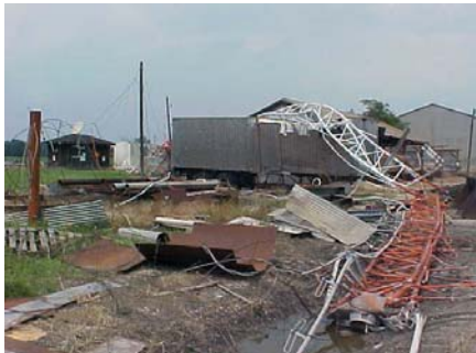
Communications tower destroyed by Katrina in southern Mississippi. (MEMA photo)
